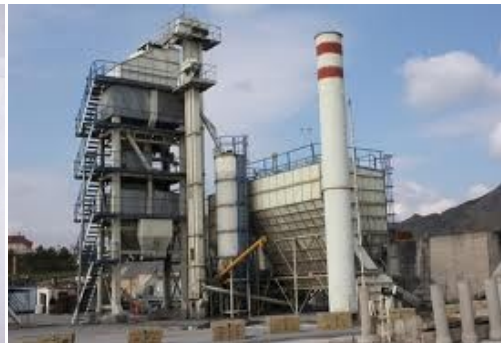
Figure 2: Asphalt plant on the site
