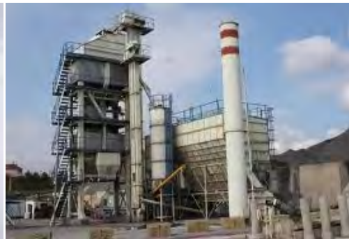
Figure 2: Asphalt plant on the site
