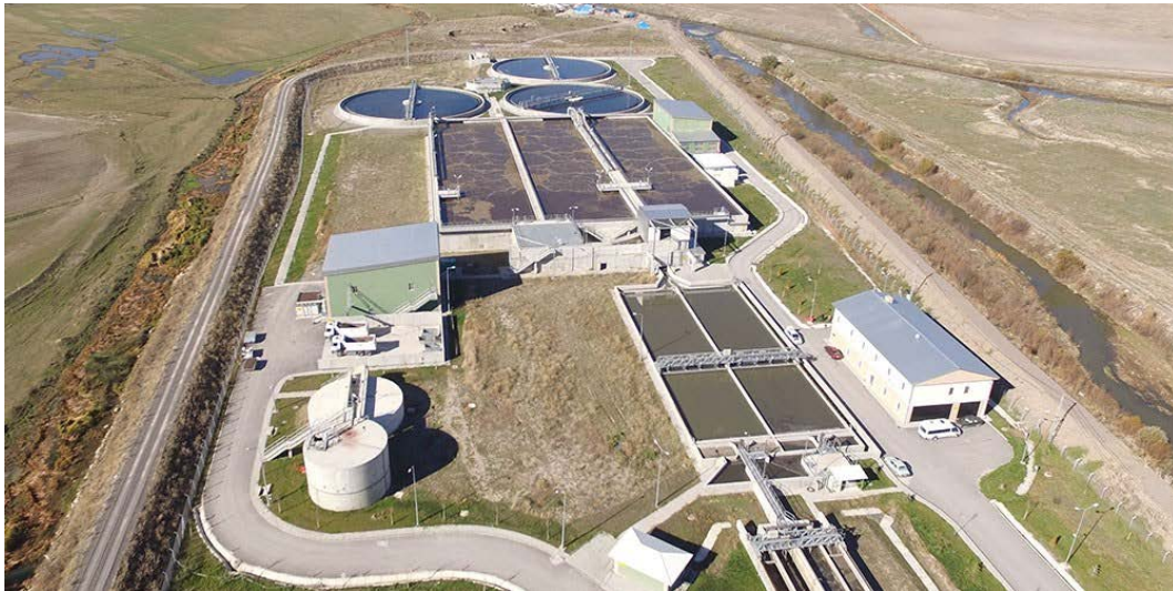
Figure 2. Erzurum Biological WWTP, 2022.
