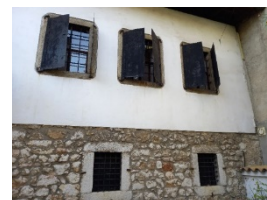
Figure 7. Iron window shutters on windows (Authors, 2022.)
