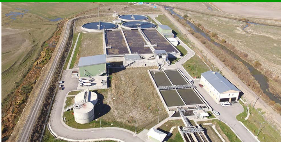
Figure 2. Erzurum Biological WWTP, 2022.
