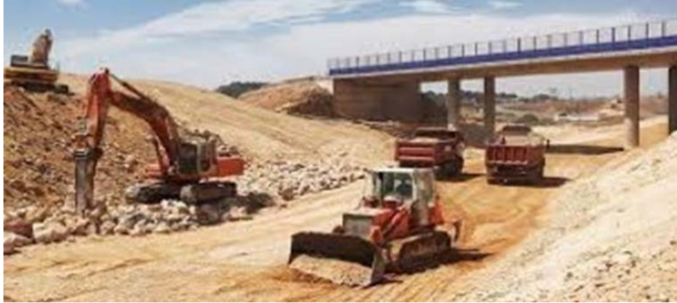
Figure 3: An example road construction site
