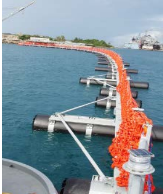
Fig. 5 Port / Harbor Offshore Barriers.[18]
