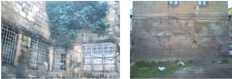
Figure 3. Examples of darkening due to air pollution in building stones
