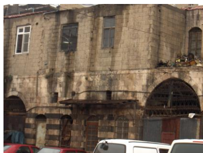
Figure 2. Examples of darkening - color change on the surface of a building
