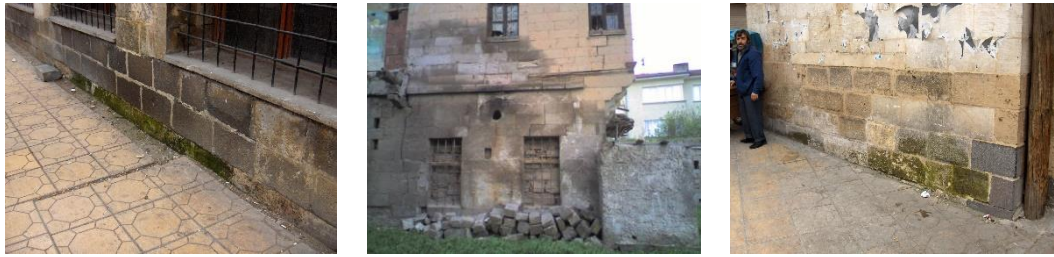
Figure 4. Wet areas on stone surfaces: color change, crusting, salt accumulation
