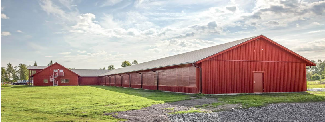
Figure 1. The Hydro66 datacenter in Boden.
