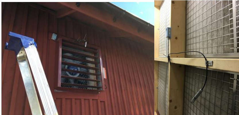
Figure 2. Sensors for measuring temperature and humidity was mounted outside the outlet fans (left part) and on the inside of the outer wall (right part) to measure the incoming air.
