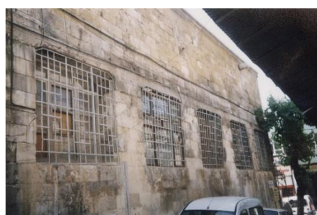
Figure 2. Examples of darkening - color change on the surface of a building
